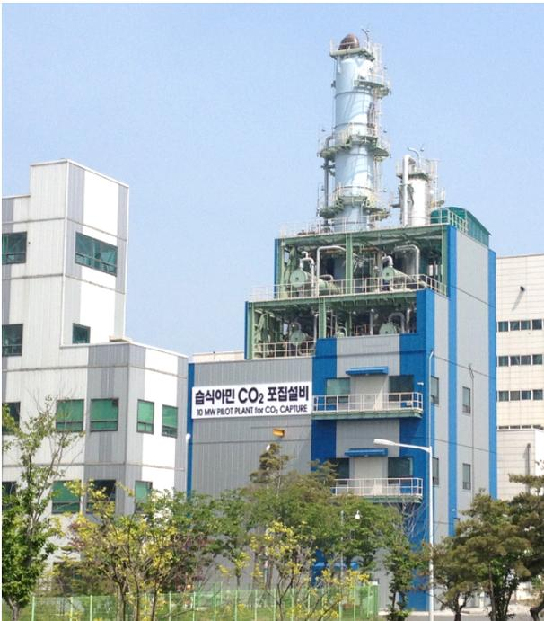
Fig. 2. CO<sub>2</sub> capture process and 10 MW wet scrubbing CO<sub>2</sub> capture plant (KOMIPO).
