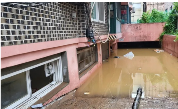
(b) Flooded semi-basement house in Gwanak-gu
